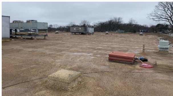
Existing Foam Roof
